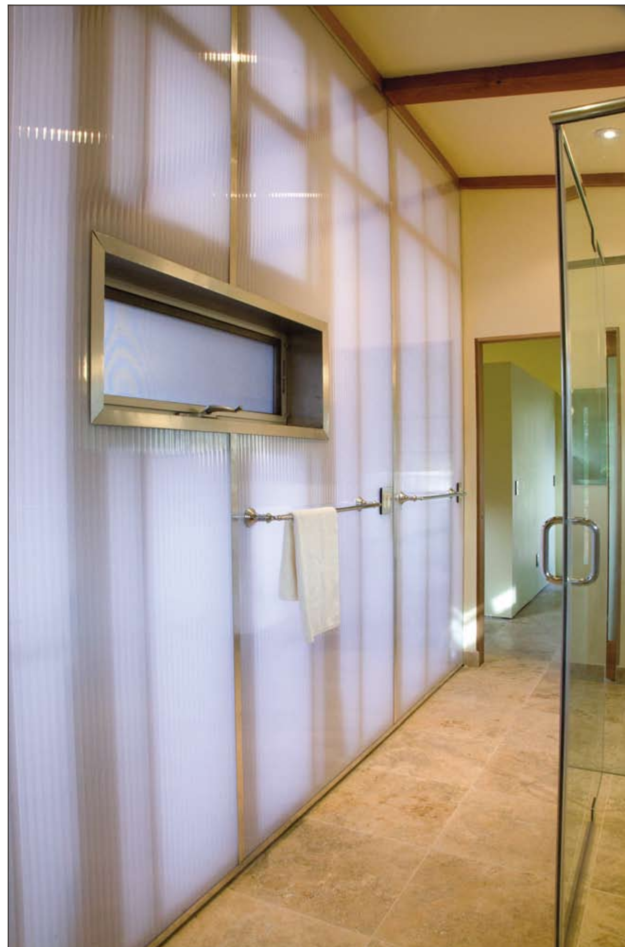
Made in Florida and obtained from a company on Oahu, polycarbonate panels are durable, lightweight and affordable. Travertine flooring from Bella Pietra inspires a spa-like ambience. Extra-wide doors and hallways are wheelchair accessible.
