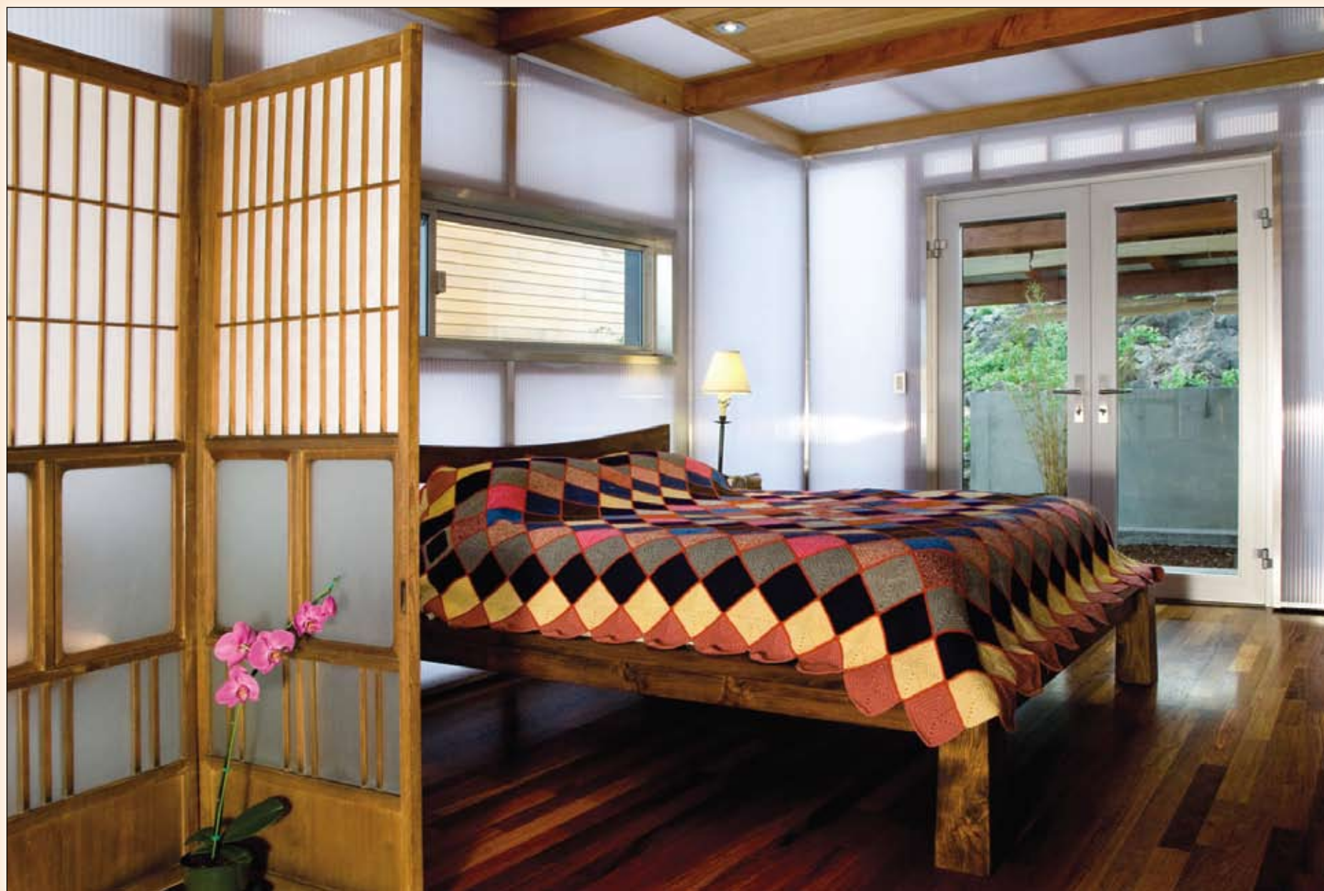
In the master bedroom, Brazilian teak flooring and unfinished cedar ceiling and walls juxtapose with polycarbonate paneling, glass and aluminum to create an organic feeling while allowing for as much light as possible. Fleetwood doors open up to a private courtyard with Japanese bath (furo).
